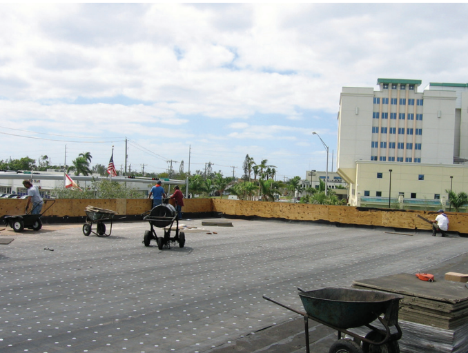
USA Roofing installing a 3 ply modified roofing system, Proper installation consist of using proper fasteners, drainage, insulation and ventilation are the key success of a flat roofing system
