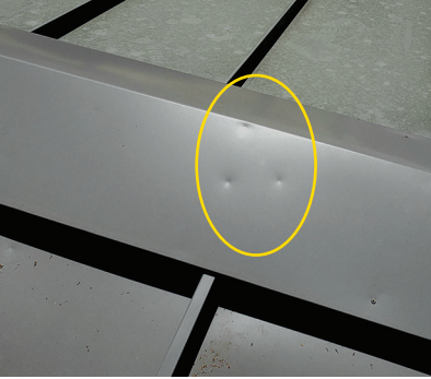
Standing Seam Damaged by Hail
