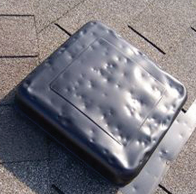
Even very small hard hail will cause damage to your roof
