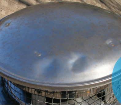
Soft metal vents will dent and show you have hail damage on your roof
