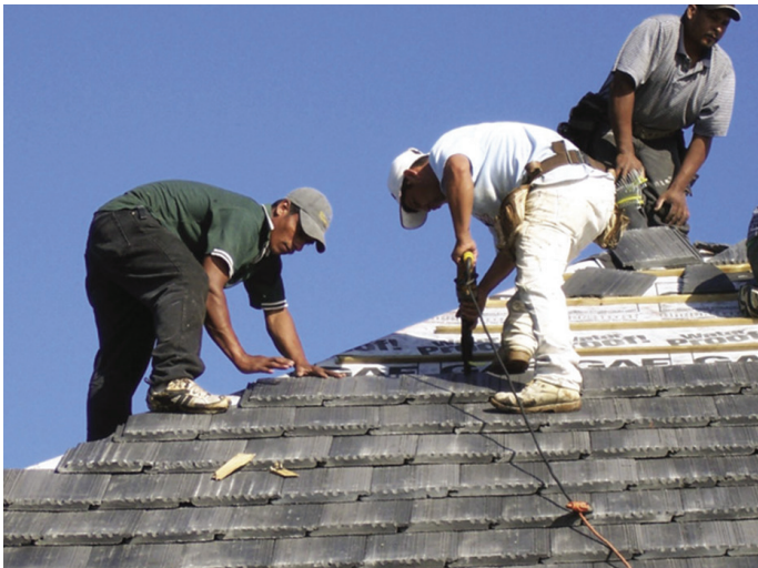
USA Roofing installing a flat concrete tile roofing system, Proper installation consist of using proper fasteners, underlayment, batten boards, spacing, and mortar.
