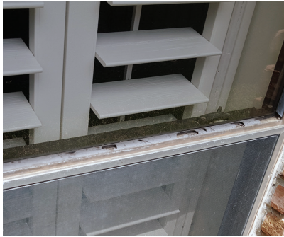
Window, trim, and screens damaged by hail
