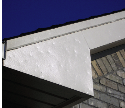
Facia, gutters siding can be damaged by hail
