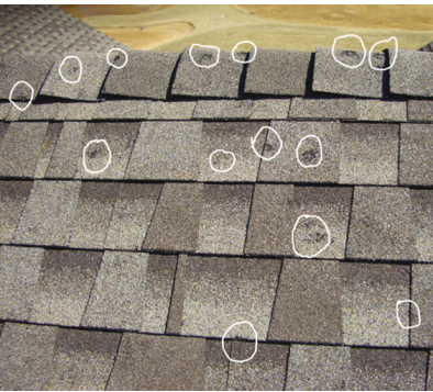
A properly inspected roof will have chalk marks to show the damage on your roof. Hail spots may be very small
