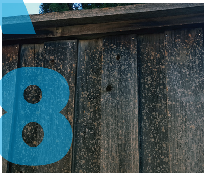
Hail damage to fences, should be pressure wash with chemicals and stained, some cases the fence has to be replaced
