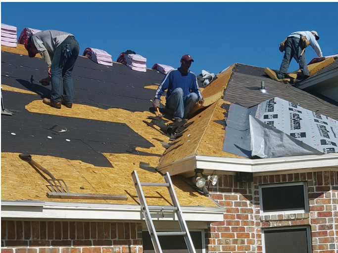
Key success of all roofing system, is using great reliable roofers, preparation of the decking, base felt, proper fasteners, proper exposure, and proper spacing.
