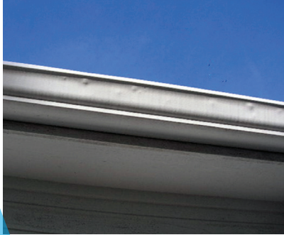
Hail can damage your gutters, downspouts and gutter screens
