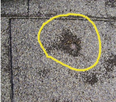
Hail hits after exposure to UV will deteriorate and expose the fiberglass felt creating leaks at a later date
