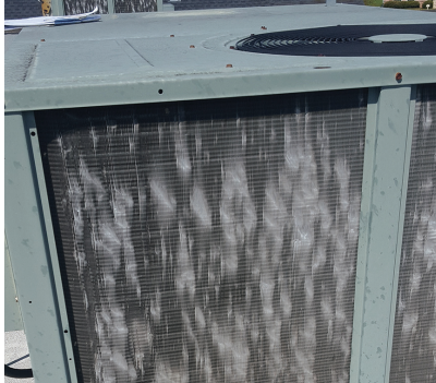
Hail can dent your Air conditioners fins and change the efficiency of your AC unit. Sometimes the unit needs to be replaced
